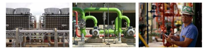
Cooling towers are used as part of industrial HVAC systems to remove heat from process water by evaporative cooling. When evaporative cooling can occur is based on local environmental variables that can be provided by one measurement: outdoor wet-bulb temperature.
