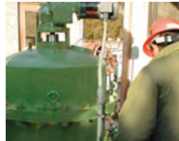
Eaton automatic strainers provide filtration of 100 micron and above. They are the perfect solution for the protection of plant equipment including spray nozzles, pump seals, water reinjection systems, water recycling systems, etc., in wastewater plants.
