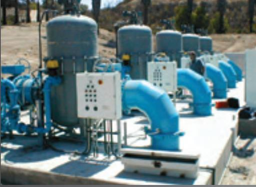
Five 24" Eaton Model 2596 units with backwash assist pumps installed at a waste water treatment plant.
