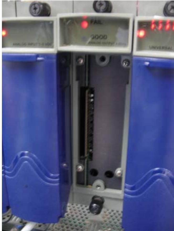
*Figure 5-9. New I/O Module in Place Prior to Attaching Terminal Board and Terminal Housing Assembly*
