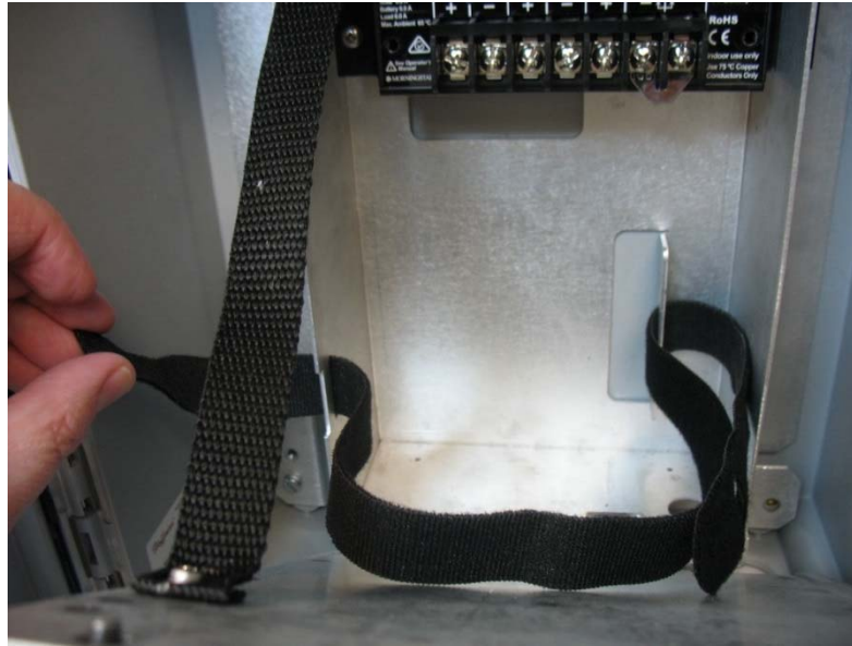
Figure 5-14: Threading the Battery Strap
